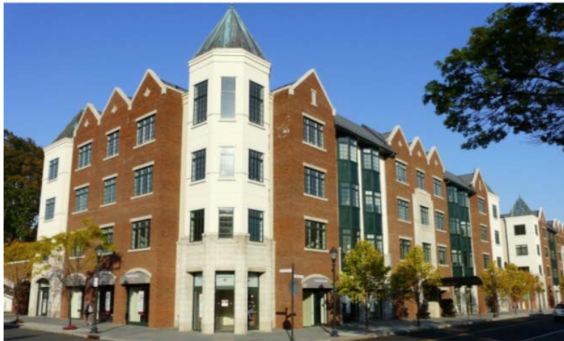
Figure 14: Christie Place (built 2008) in Downtown Scarsdale
