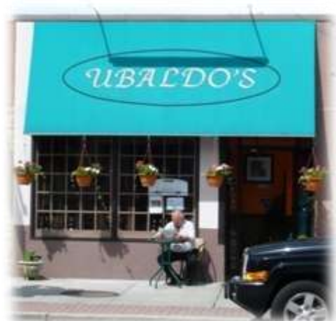
While fabric awning signs such as this present an attractive image, they can hide important architectural elements and provide little effective shade. Shallow awnings like this contribute little to the pedestrians' sense of enclosure along the street. Traditional awnings should be preferred.
