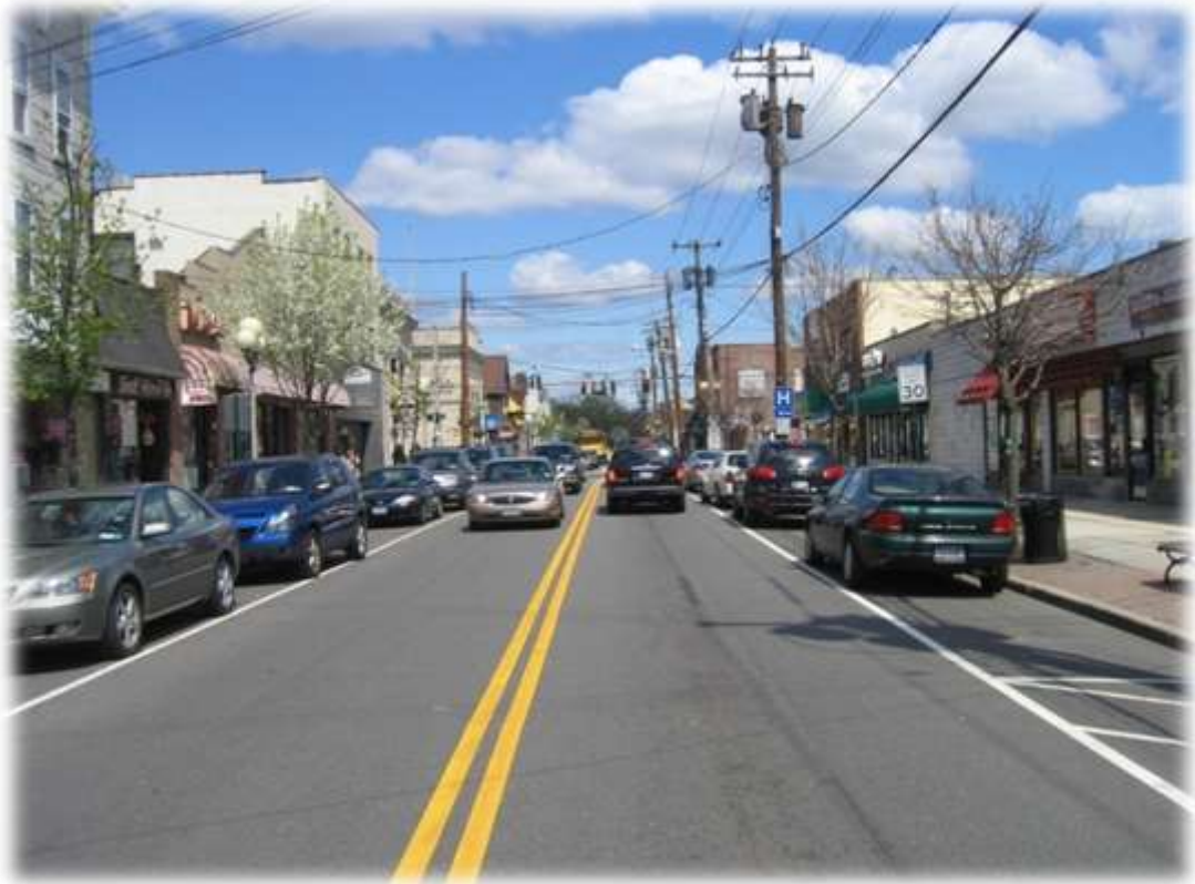
Typical section of Main Street in the downtown area, which is a two lane undivided roadway with parallel parking available on both sides.
